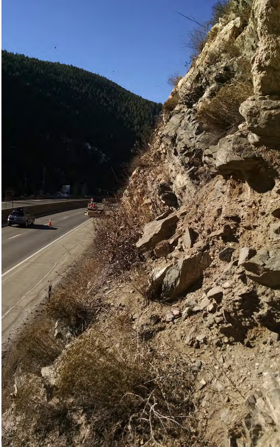
Photo 3 – Existing (looking) Westbound rock cut with colluvium deposits. Note cobbles and boulders.
