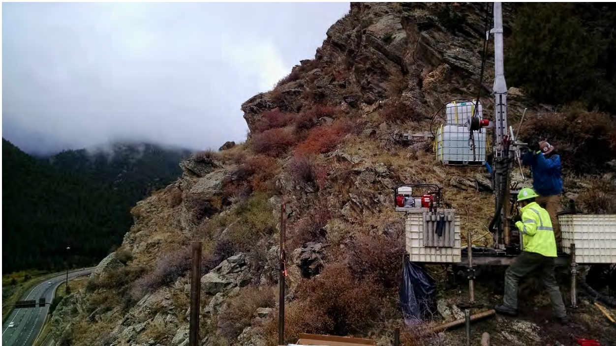
Figure 5. Bedrock structure at East Portal boring YA-EP-1 (looking West).
