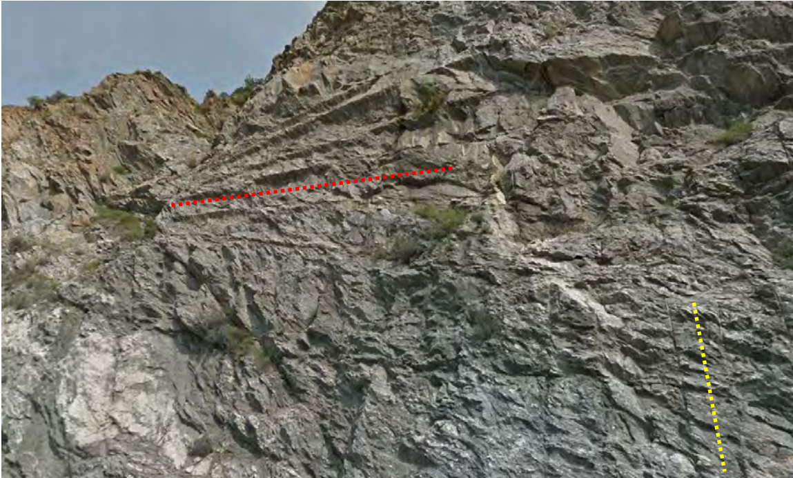
Figure 3. Existing rock cut, vertical (yellow) and fan-drilled (red) half-casts.
