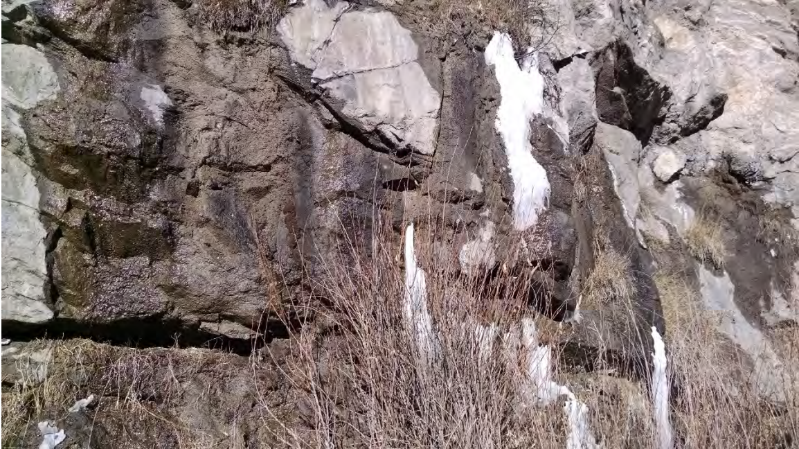
Photo 1 – Ice and springs from water seeps; localized and not representative of the rock cuts.
